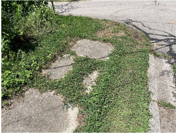
Figure 10: Sidewalk in poor condition
