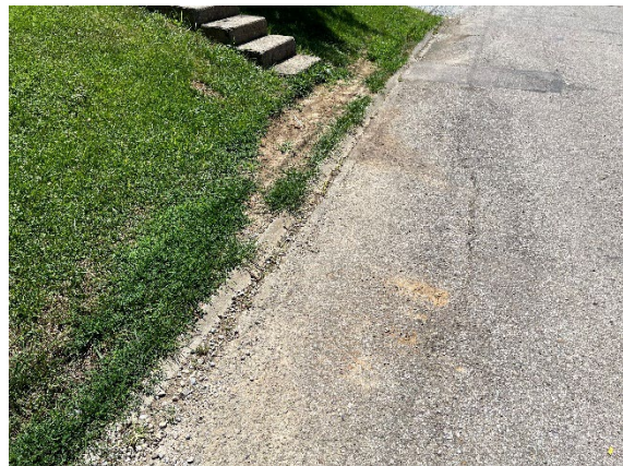
Figure 11: Curb in poor condition
